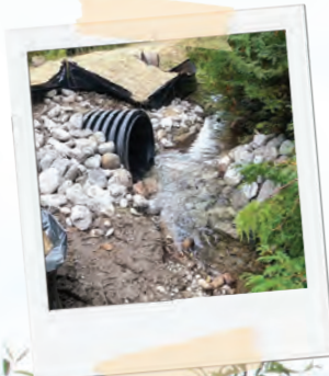
Lowered culvert to reconnect coldwater stream.
