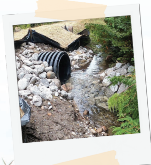
Lowered culvert to reconnect coldwater stream.
